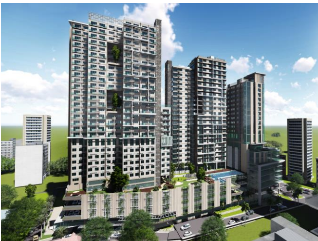
Base Line Prestige is a 351-unit residential condominium along Juana Osmena Street in Cebu City.
